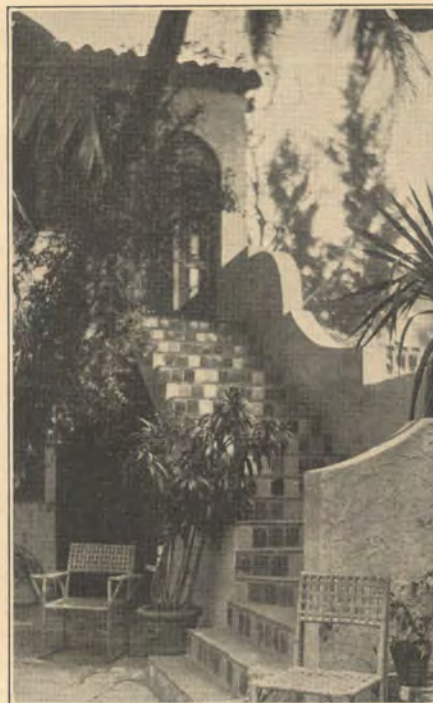
This stairway shows a use of Mizner tile. The risers are in variegated colors.
