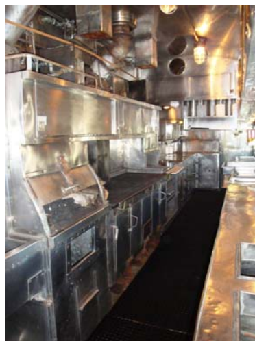
The kitchen, after restoration. Photo by Clay Wieland
